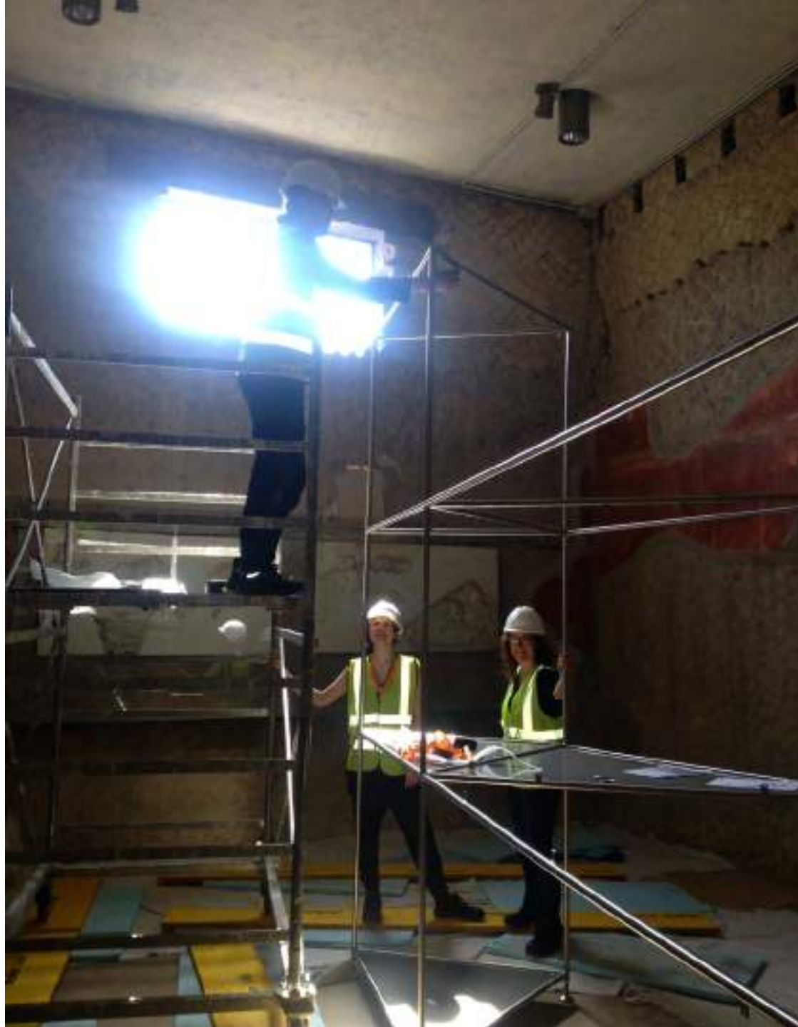
Installation process of Expanded Interiors at the House of the Beautiful Courtyard, Herculaneum
